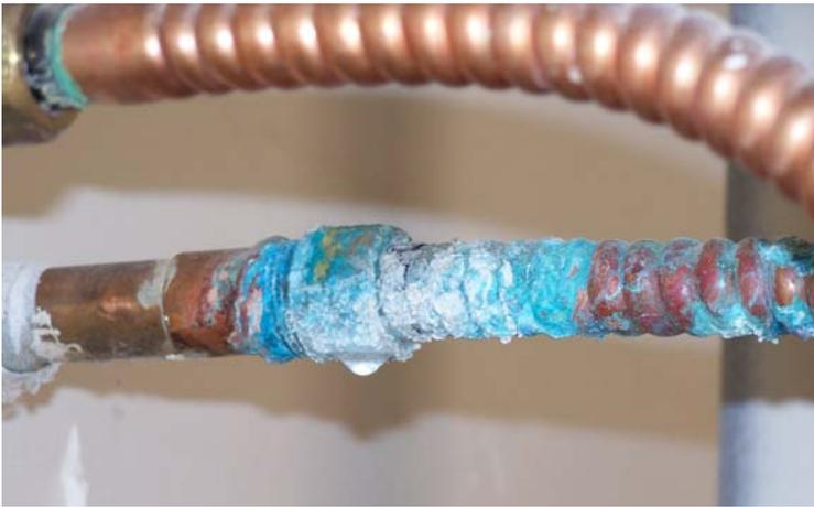
Figure 1. Corrosion at a connection on a water heater indicated by the blue-green color.
